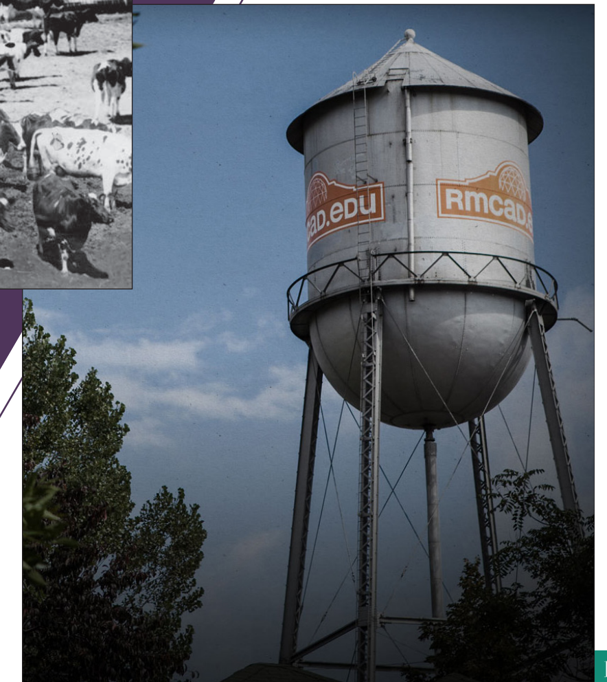
Rocky Mountain College of Art + Design Water Tower built by JCRS in 1910
