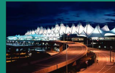
Denver International Airport
